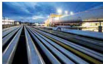
Below and right: LPG storage in Puerto Rico and Estonia.
