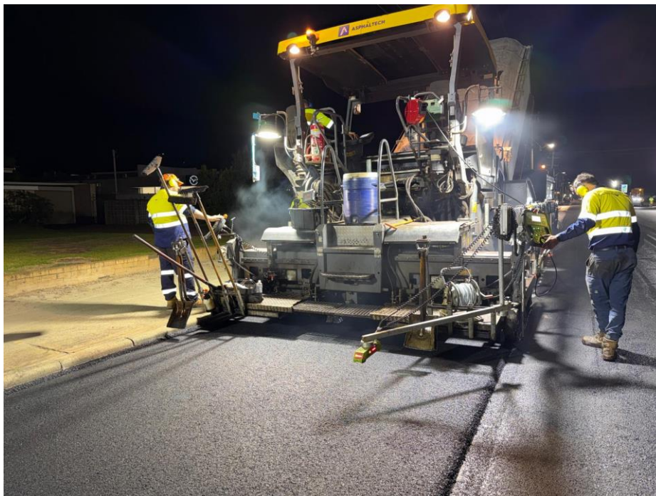
Figure 1 CarbonBind A15E Asphalt DG 10 Wearing Course
