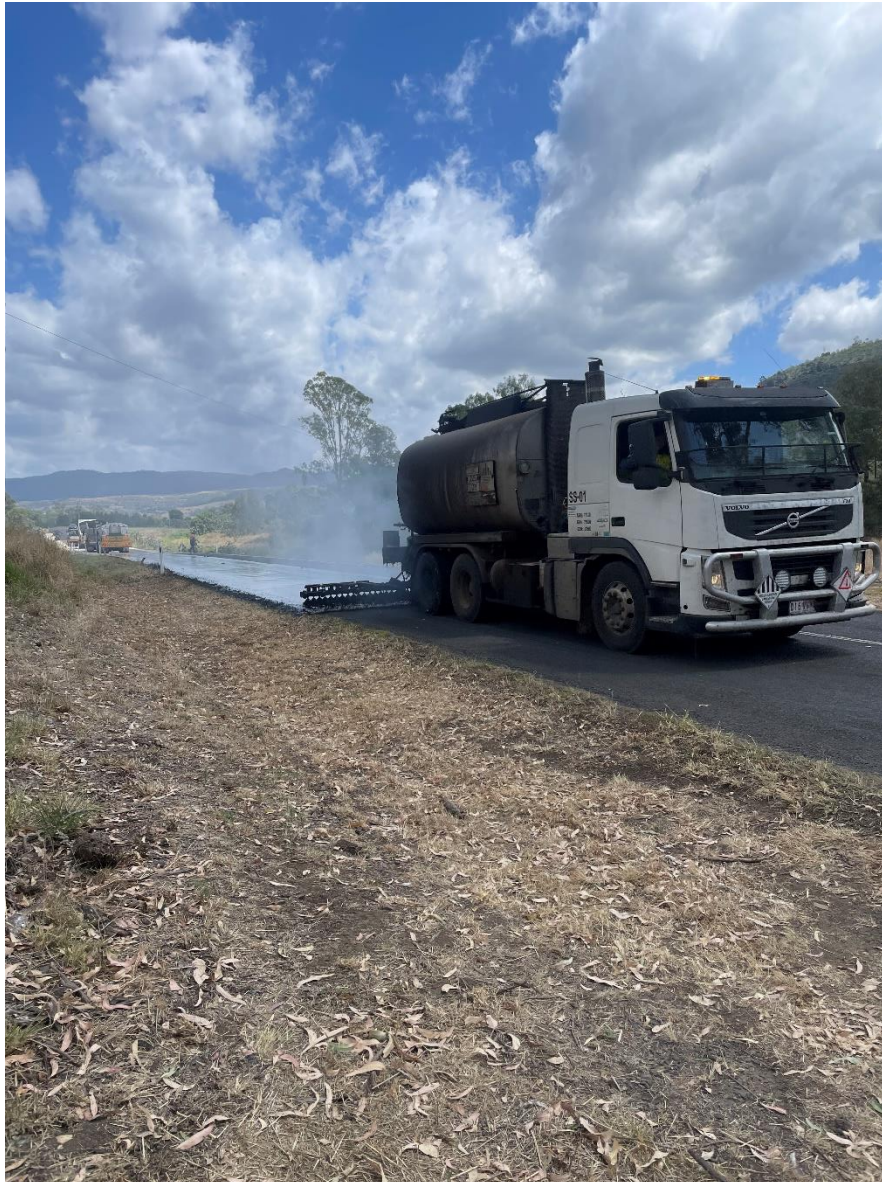
Figure 5, CarbonBind C170 being Sprayed
