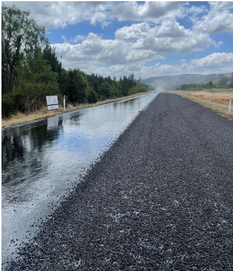
Figure 2, CarbonBind C170 sprayed on site
