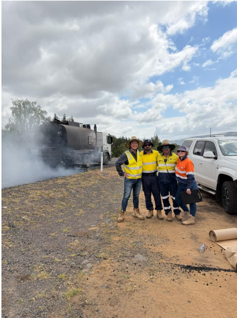
Figure 4, Site Photo of CarbonBind C170 being sprayed for the first time
