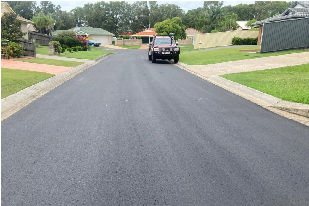
Figure 3, Image of CarbonBind C320 Laid
