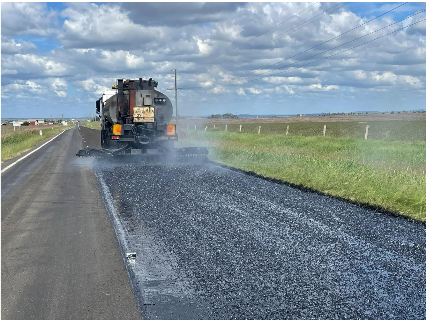
Figure 2, Spraying CarbonBind S15E
